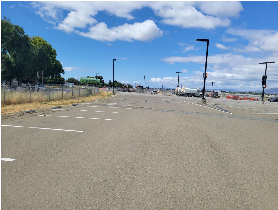
View facing north from southwest corner of Subject Property.
