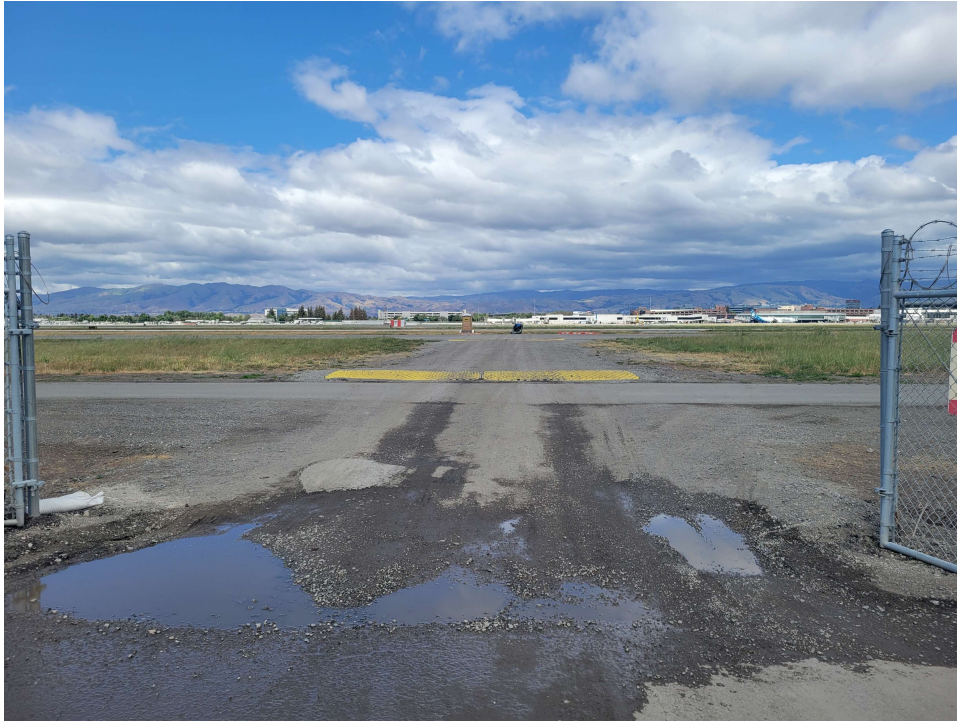
View of entrance into airfield area and Taxiway V construction zone.
