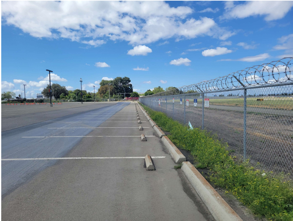
View facing north along security fence.
