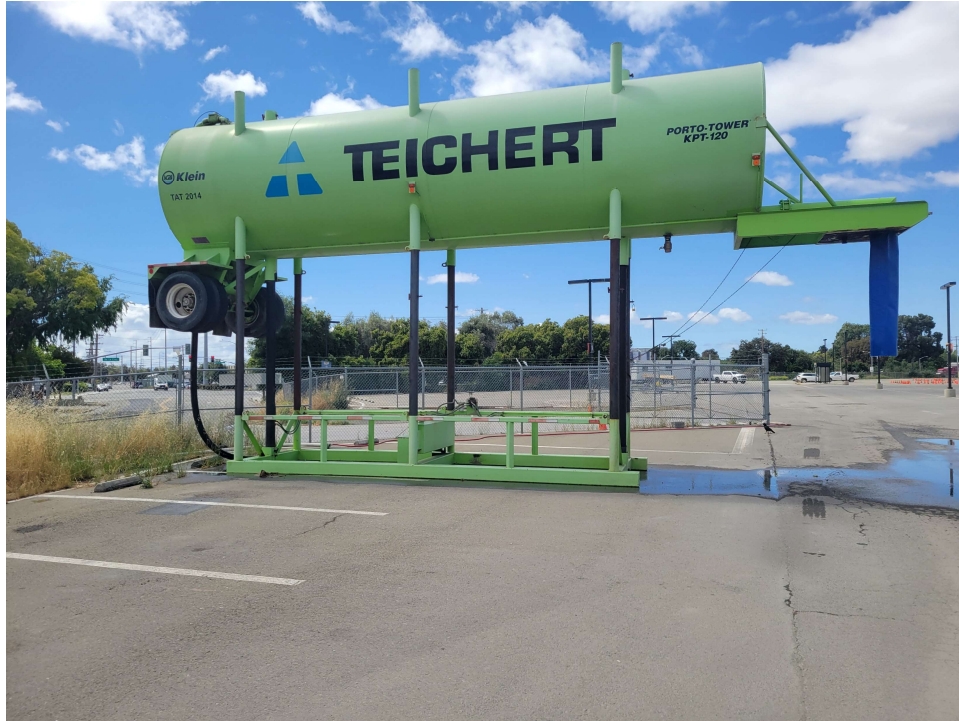
Temporary water storage associated with construction of Taxiway V.
