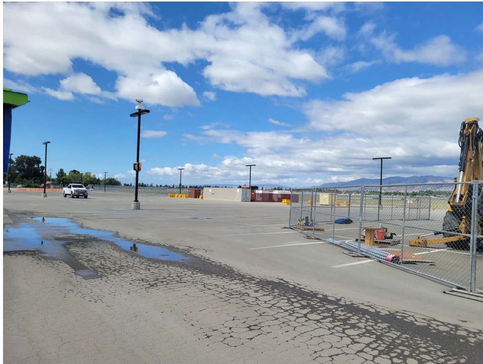
Staging area for equipment used in connection with Taxiway V construction.
