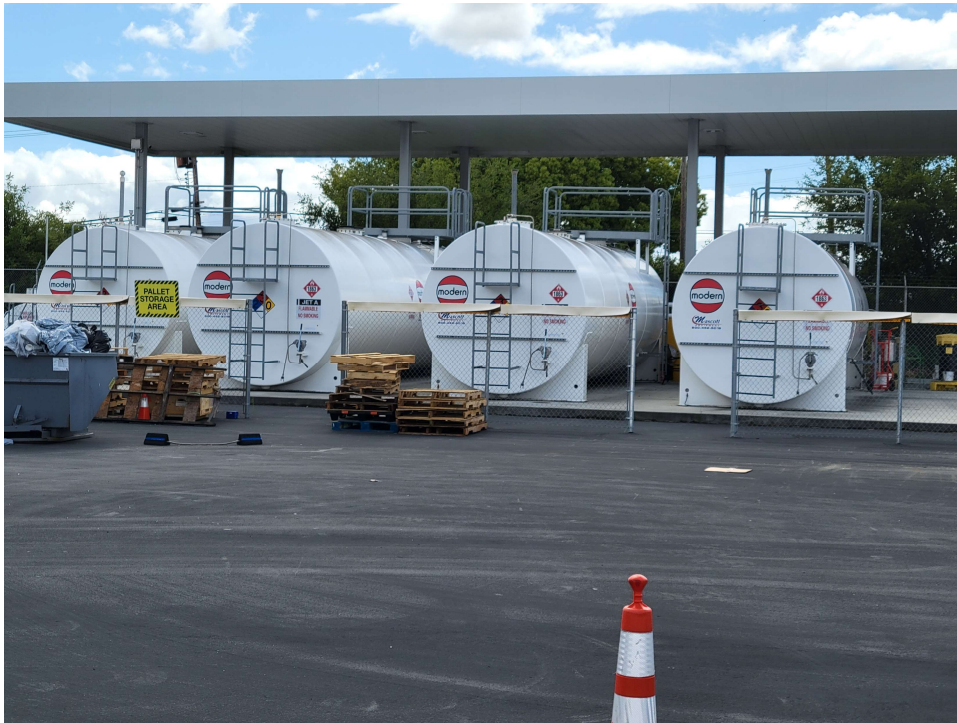
Fuel storage area located south of Subject Property.
