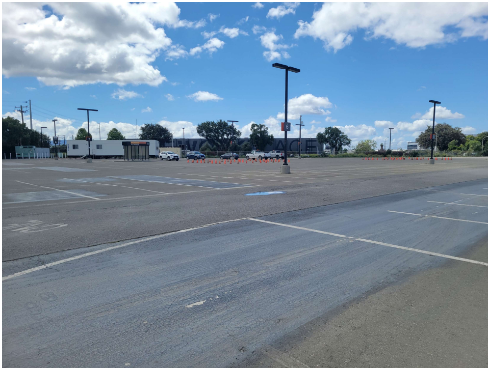
View facing west towards temporary offices staged at Subject Property.
