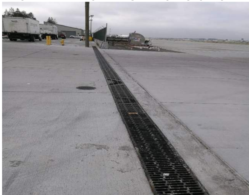
TRENCH DRAIN AT NORTHEAST PARCEL STORAGE AREA
