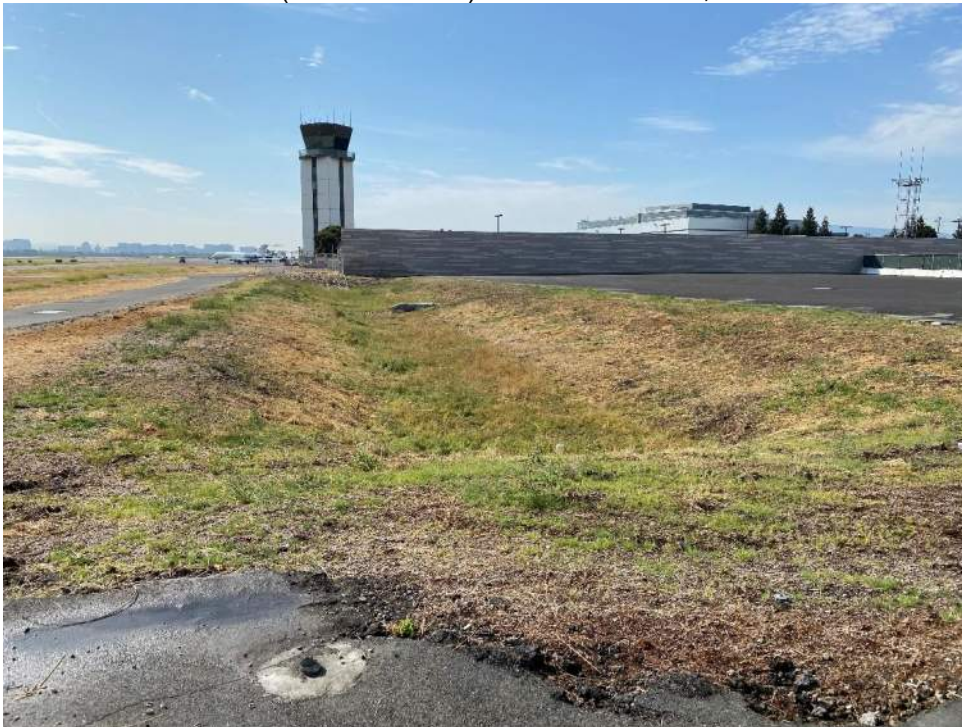
BIORETENTION CELL (SOUTHEAST) AT SIGNATURE, FACING SOUTHWEST
