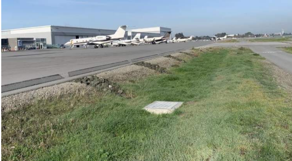
BIORETENTION CELL (EAST) AT SIGNATURE, FACING NORTH-WEST
