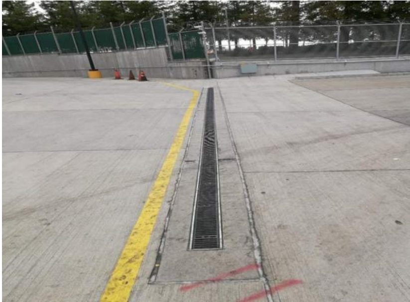
TRENCH DRAIN AT NORTHEAST PARCEL STORAGE AREA
