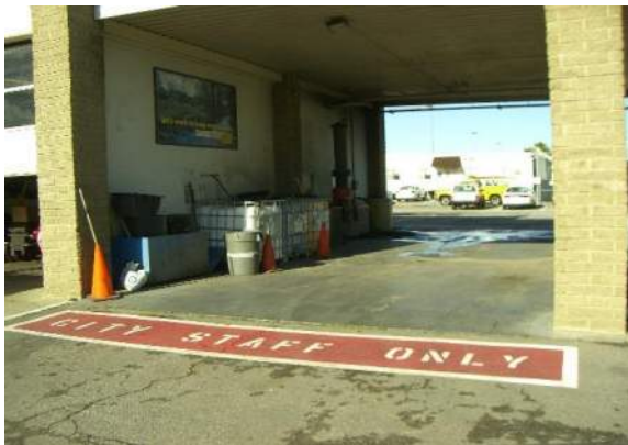
FLEET MAINTENANCE WASH RACK
