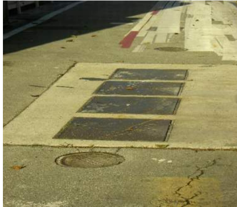
PAINT SHOP CLARIFIERS
