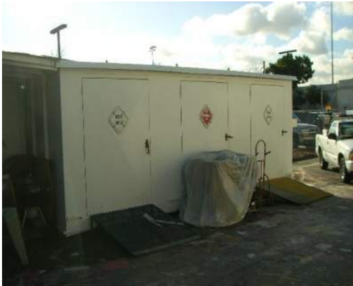
PAINT SHOP STORAGE
